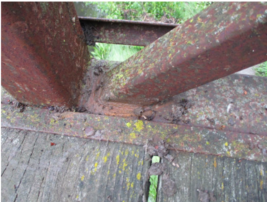
Image 6: Truss Typical Brace/Post Bottom Connection
