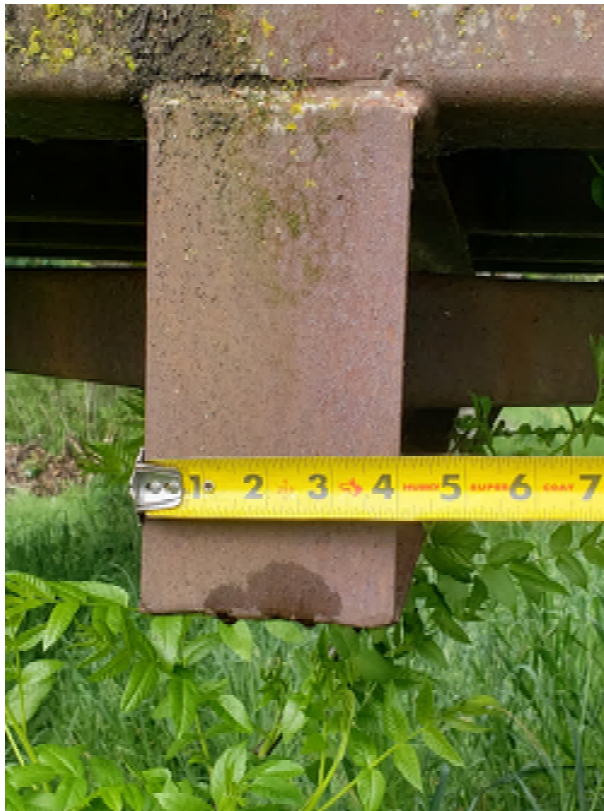
Image 10: Gravity Purlin Connection
