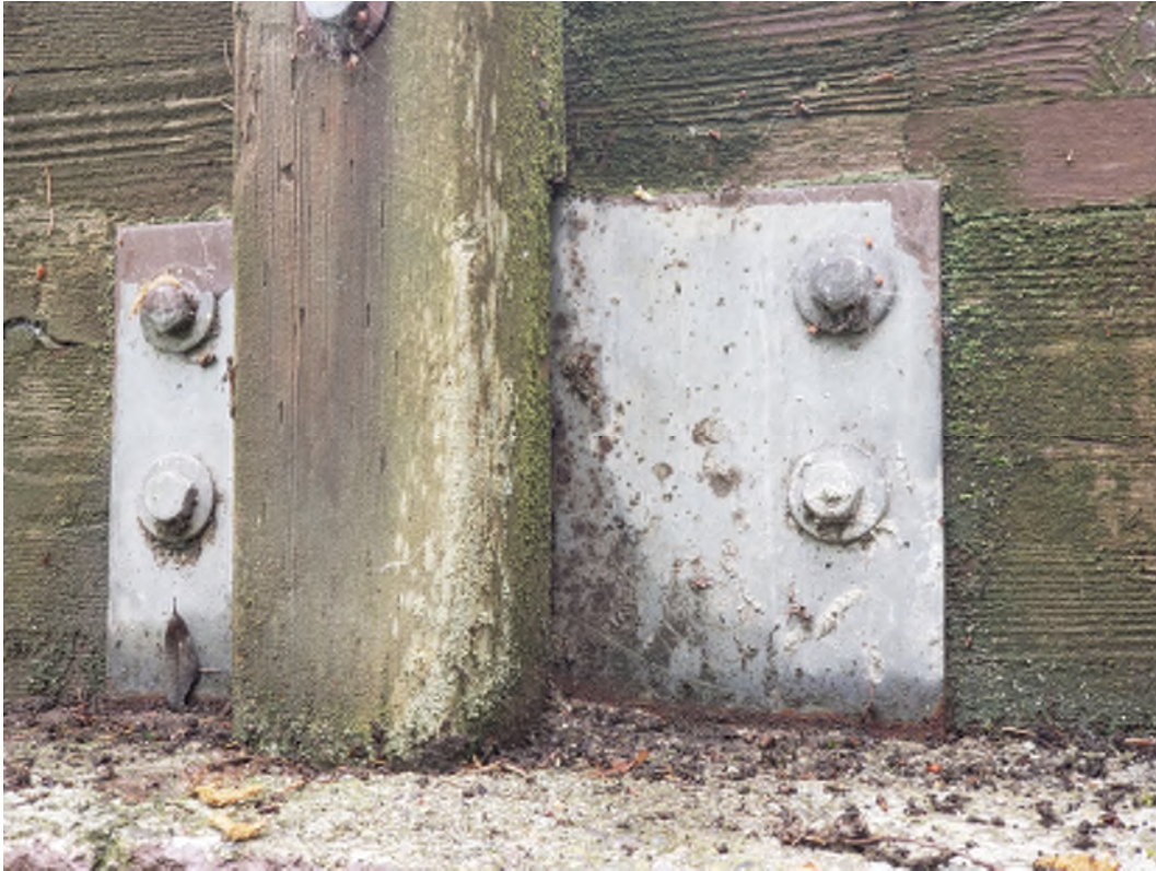
Image 11: Center Girder Splice
