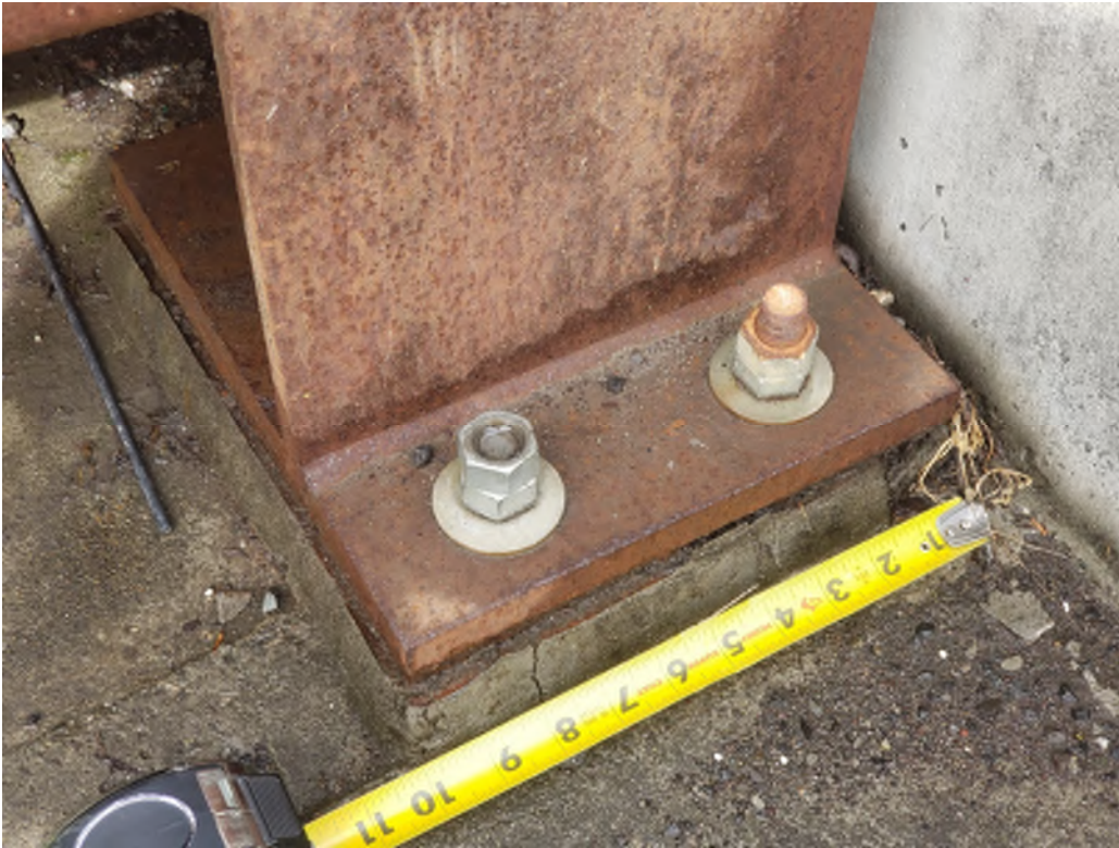
Image 8: Typical Bearing Plate and Anchor Bolt
