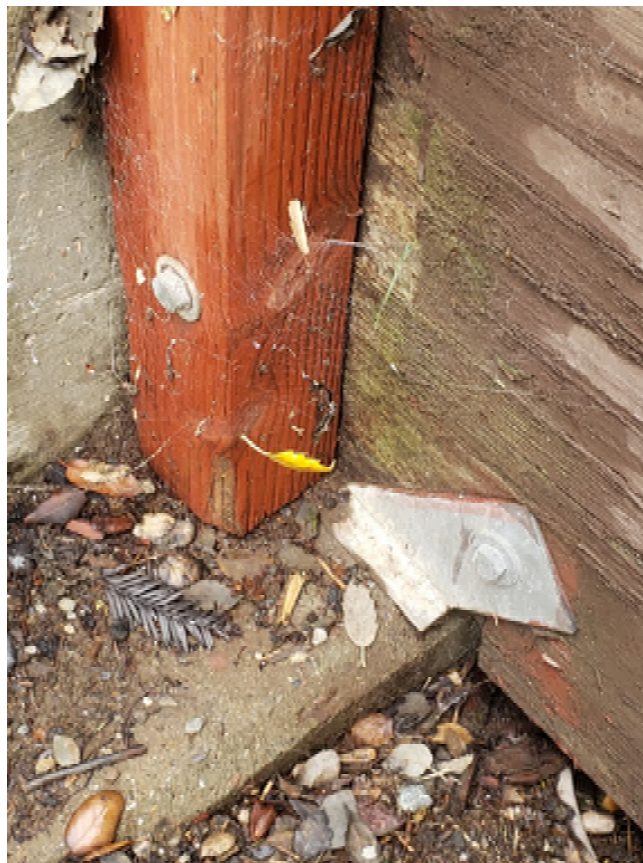
Image 10: Typical Bearing Plate and Anchor Bolt
