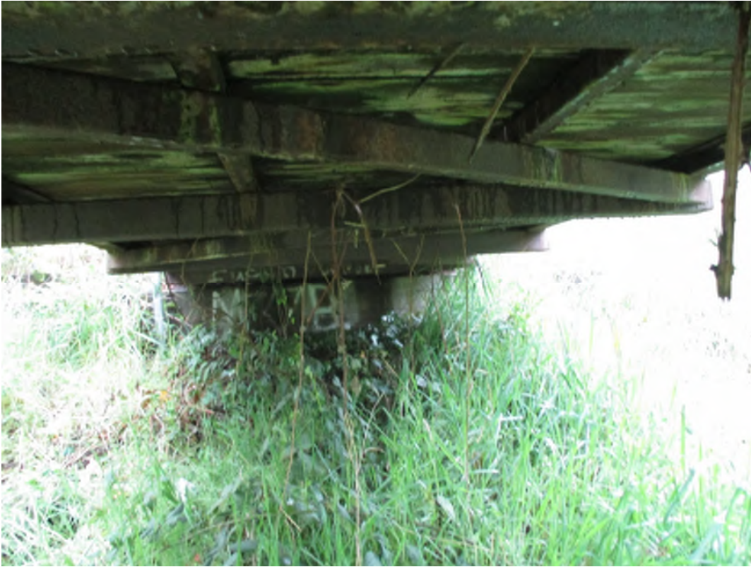
Image 13: Horizontal Truss at Underside of Bridge
