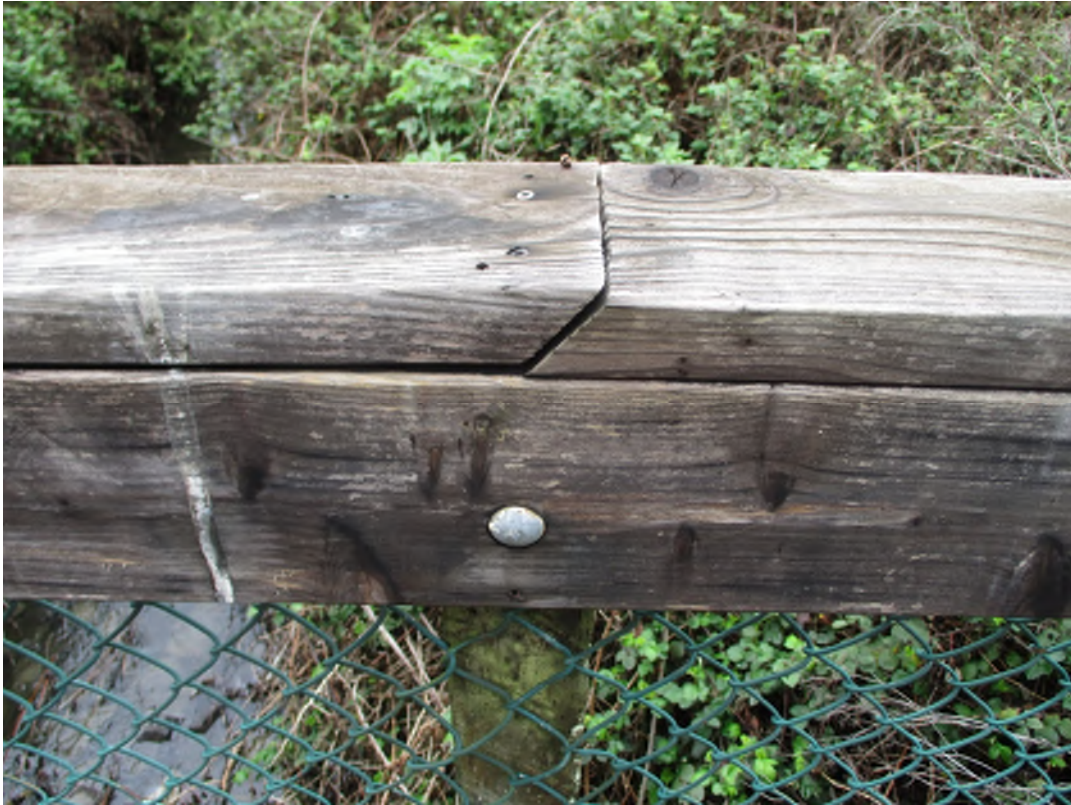
Image 7: Handrail Member Joint
