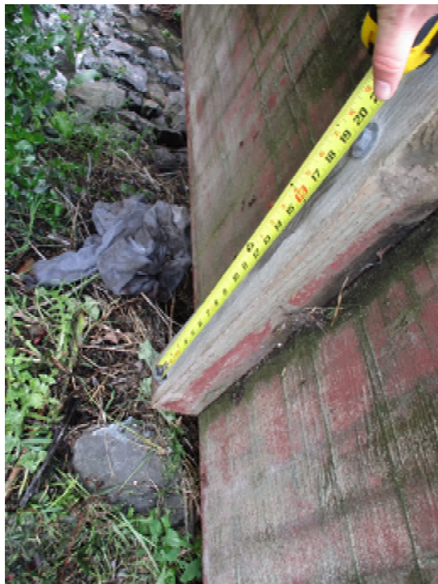
Image 6: Handrail Post Connection
