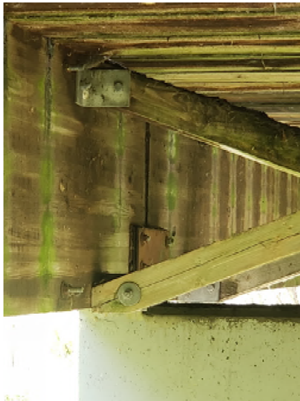
Image 14: Lateral Bracing at Center Splice
