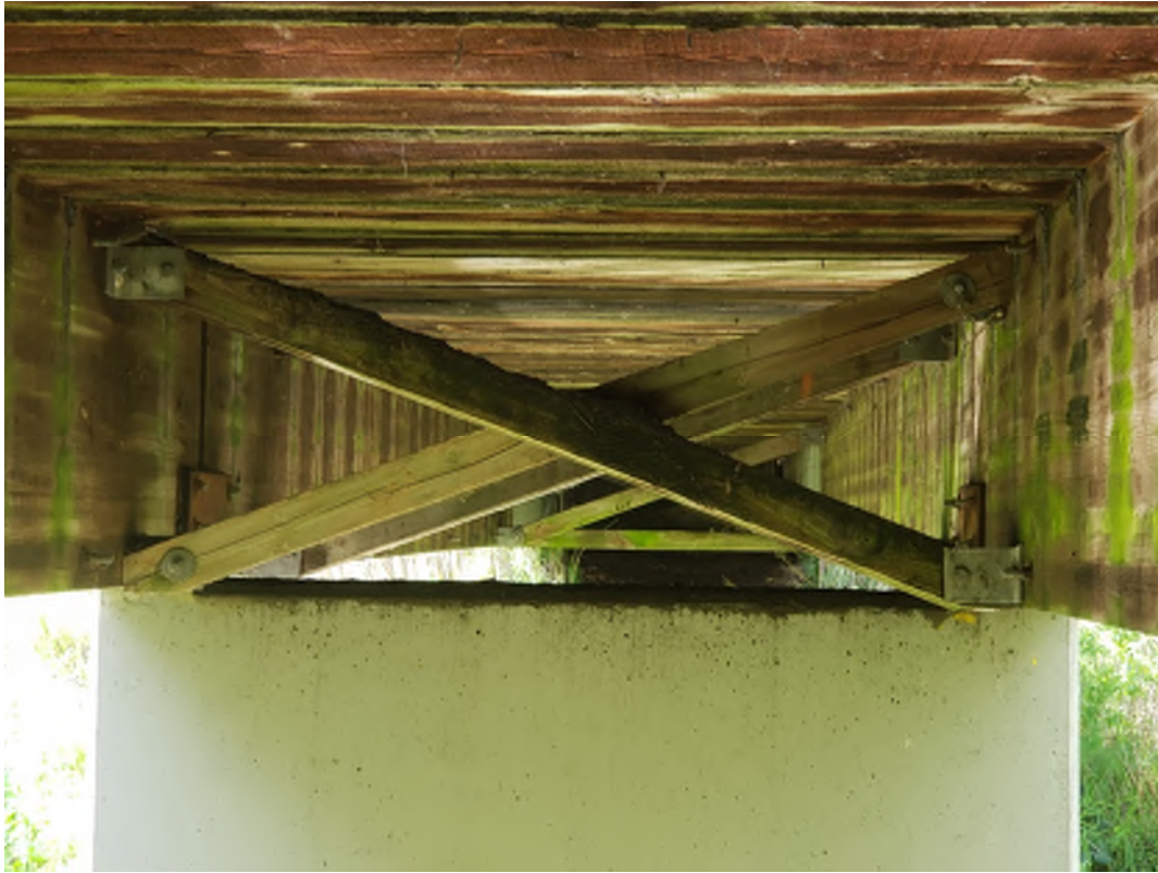
Image 13: Underside of Bridge
