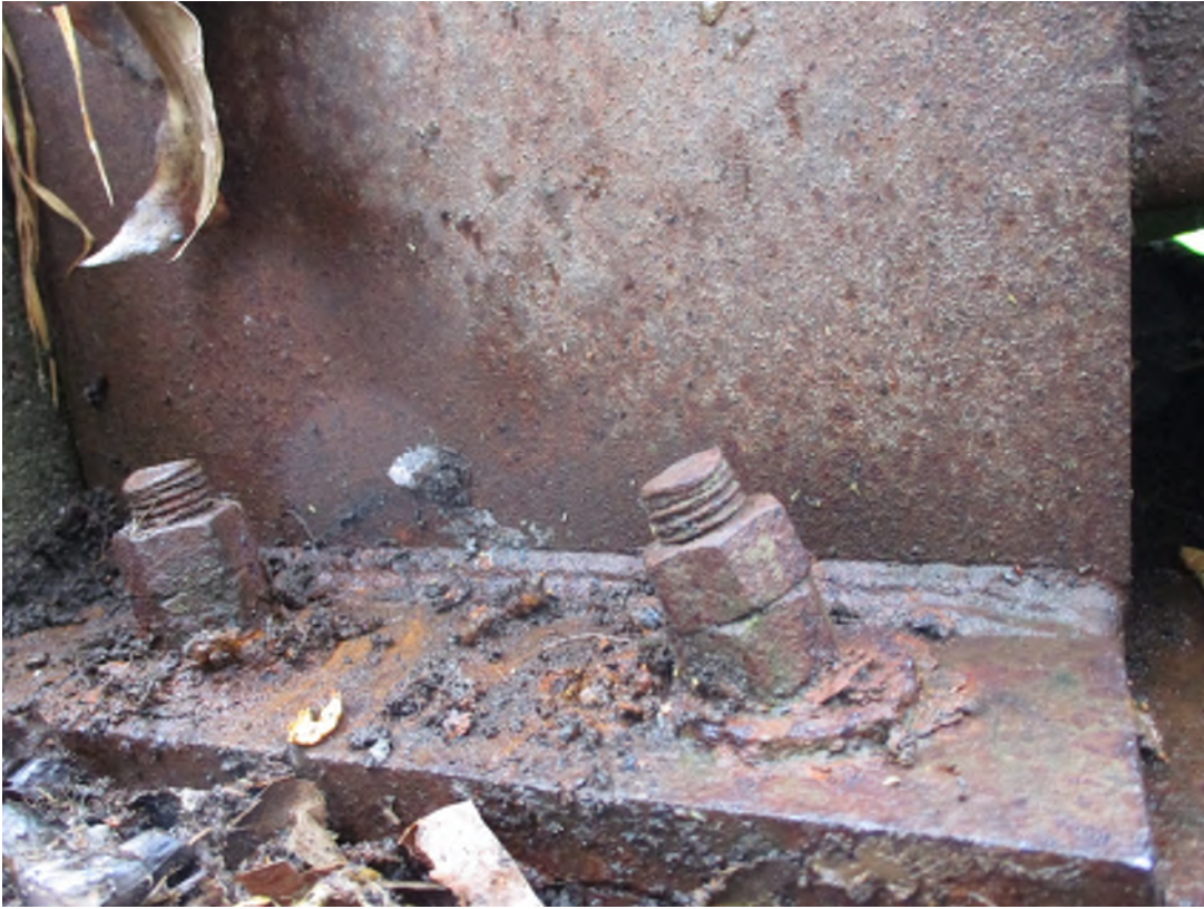
Image 11: Bearing Plate with Bent Anchor Bolts
