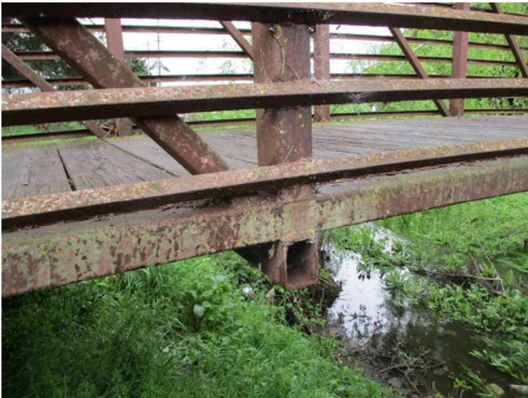
Image 12: Gravity Purlin Connection
