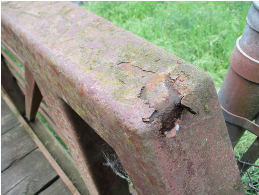
Image 12: Deteriorating Finish
