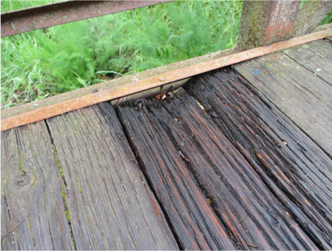
Image 9: Rotten Floorboard
