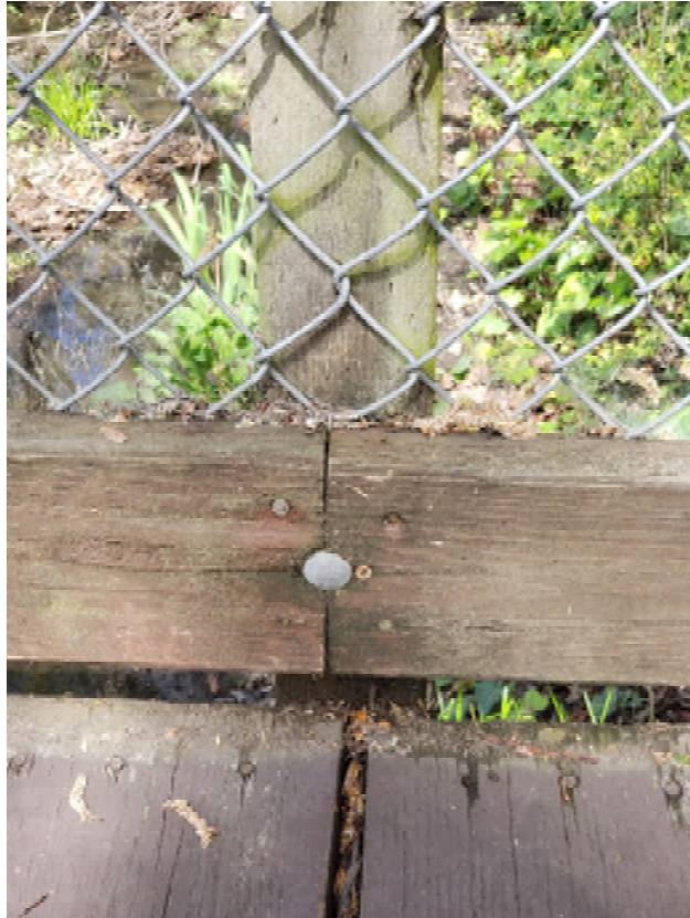
Image 7: Guardrail Member Joint
