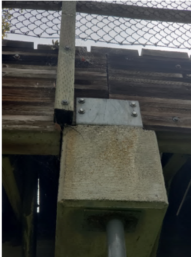
Image 11: Center Girder Splice
