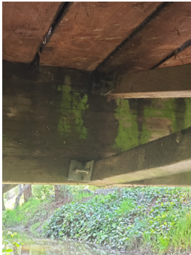
Image 12: Lateral Bracing
