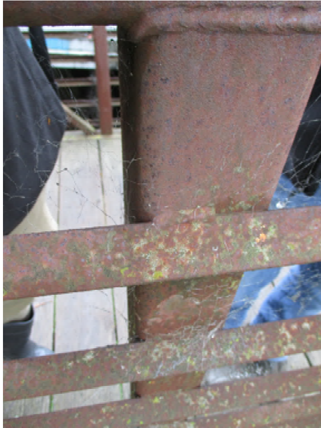
Image 7: Typical Handrail Member Weld
