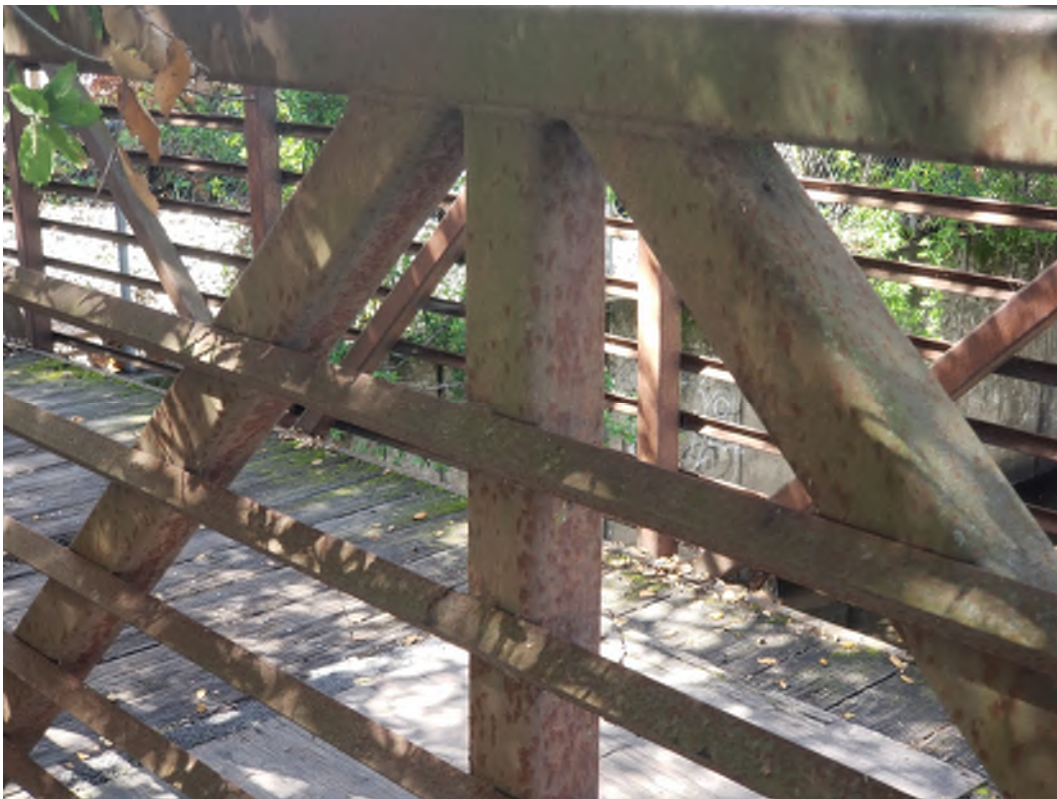
Image 6: Typical Handrail Member Weld
