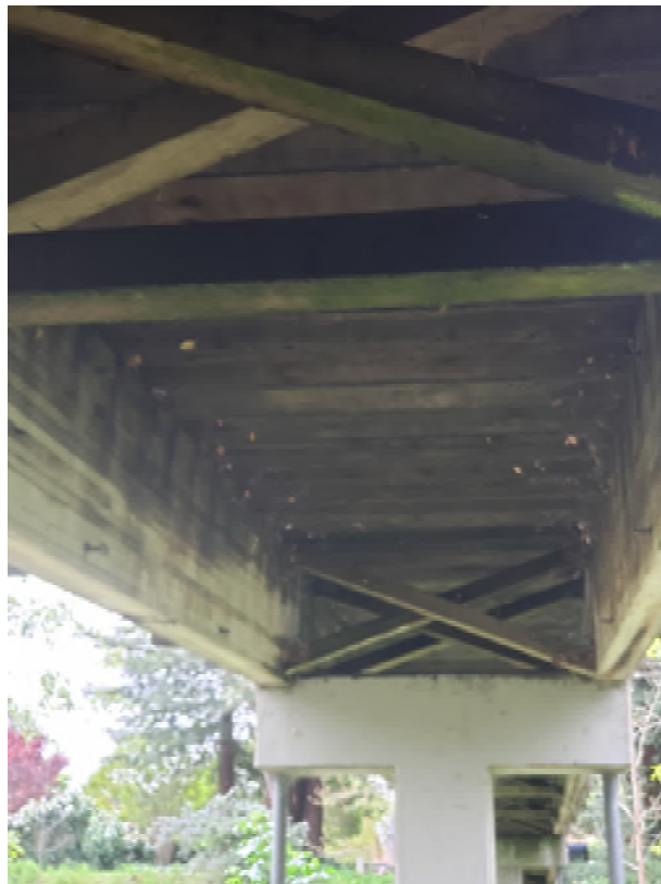
Image 14: Lateral Bracing at Center Splice
