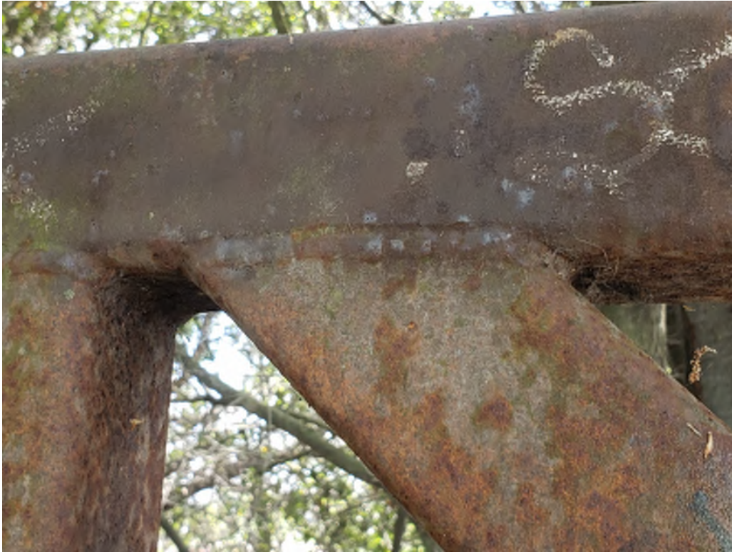
Image 5: Truss Typical Brace/Post Top Connection
