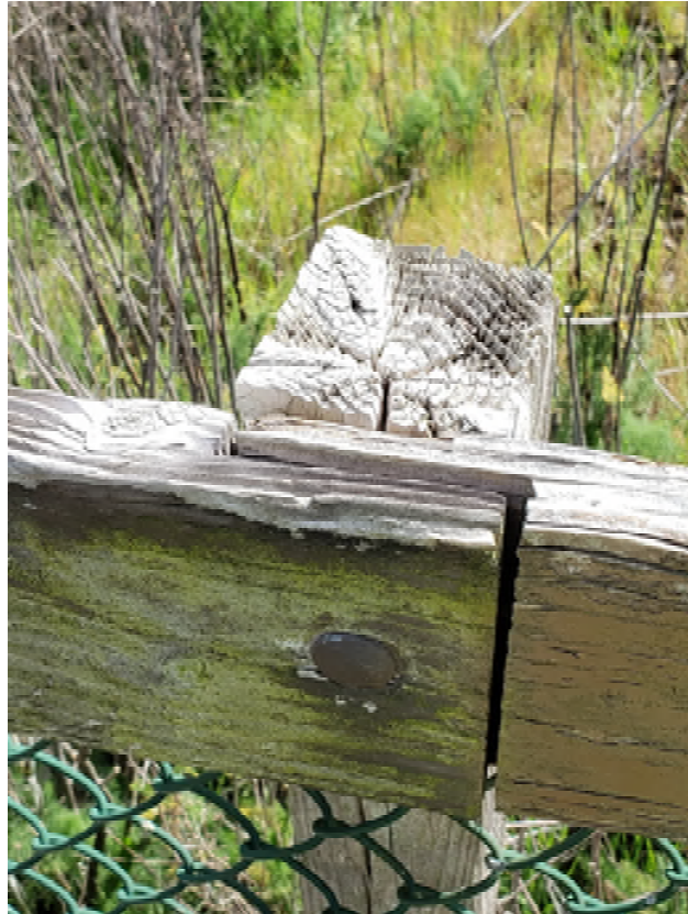
Image 7: Handrail Member Joint
