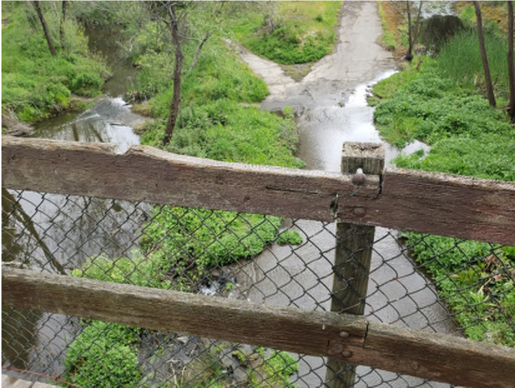
Image 7: Handrail Member Joint
