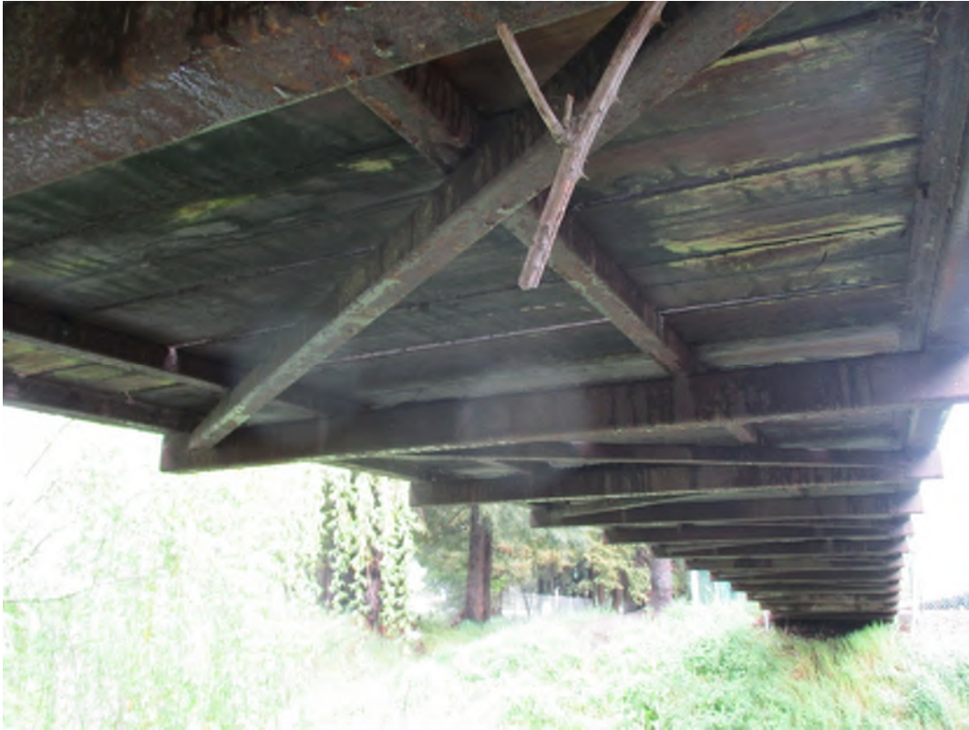
Image 13: Horizontal Truss at Underside of Bridge
