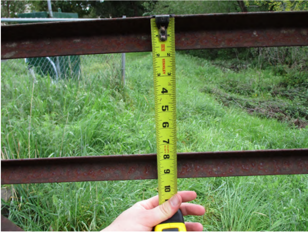
Image 15: Maximum Horizontal Member Spacing
