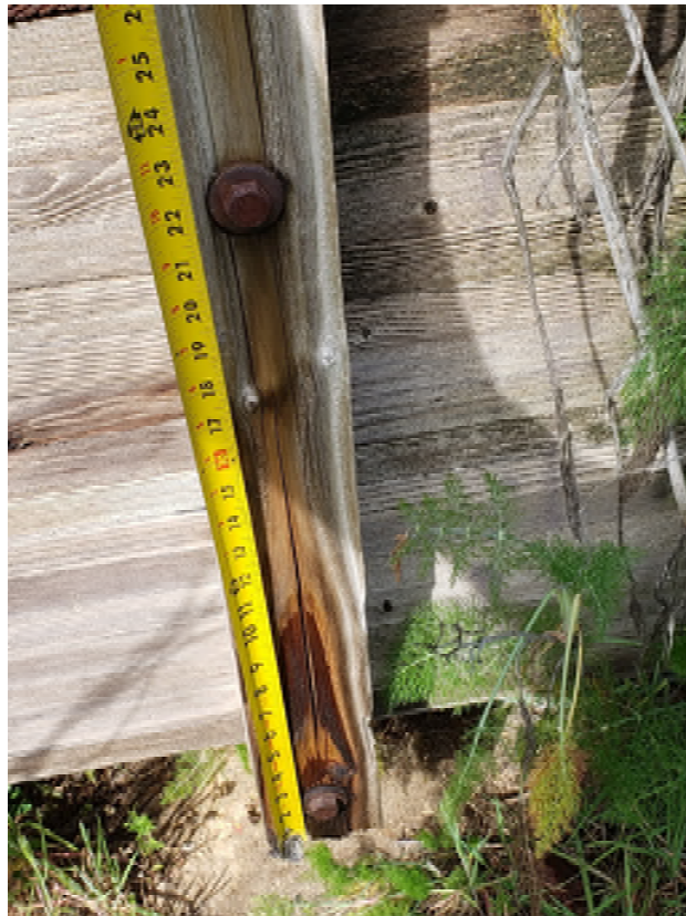
Image 6: Handrail Post Connection
