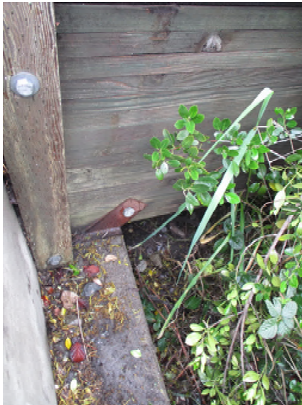
Image 10: Typical Bearing Plate and Anchor Bolt
