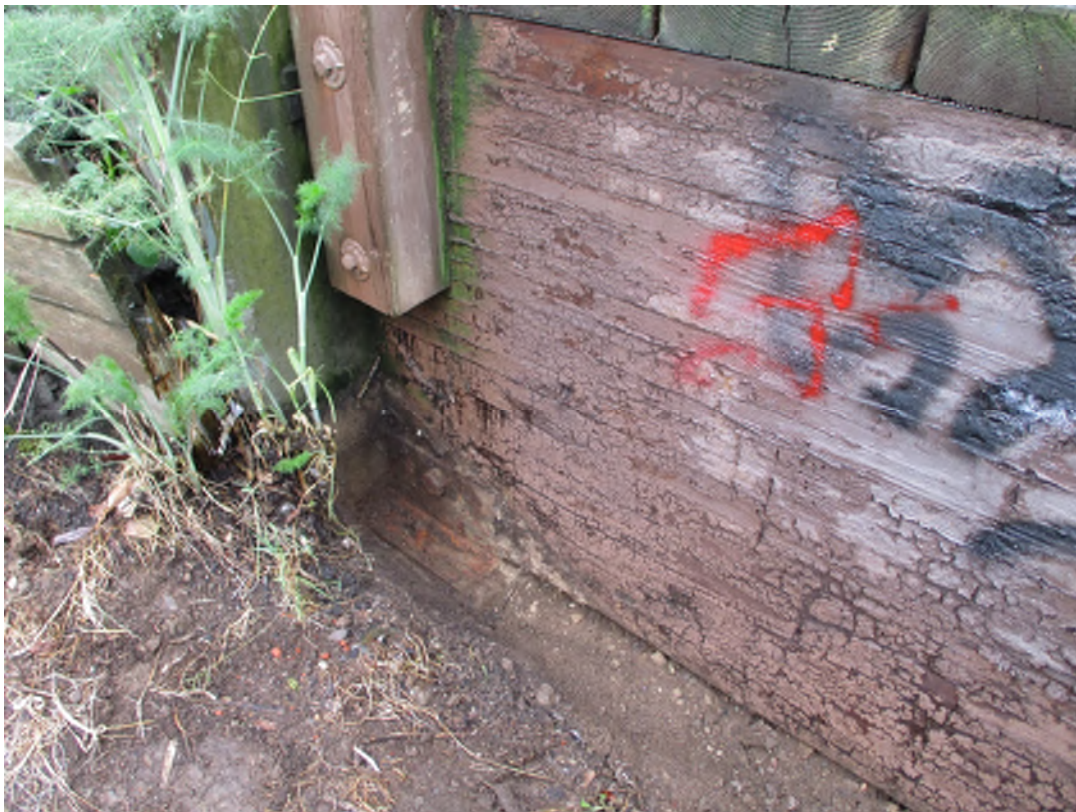
Image 10: Typical Bearing Plate and Anchor Bolt
