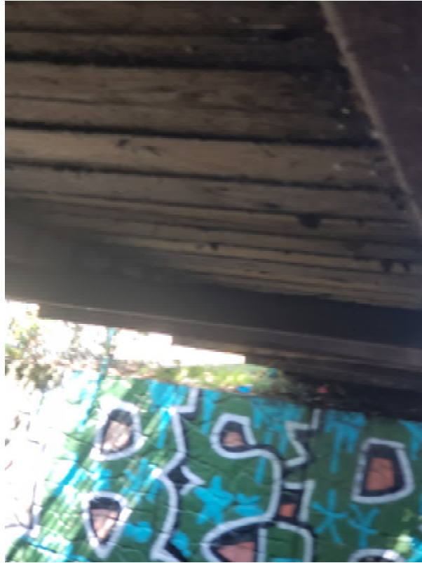
Image 13: Underside of Bridge
