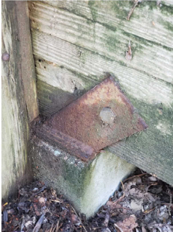
Image 9: Typical Bearing Plate and Anchor Bolt
