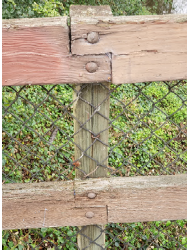
Image 5: Handrail Joints
