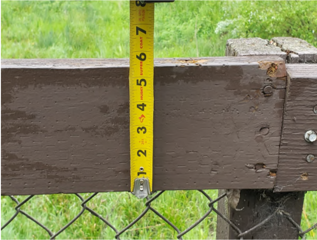
Image 7: Handrail Member Joint
