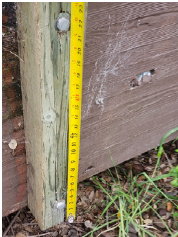
Image 6: Handrail Post Connection
