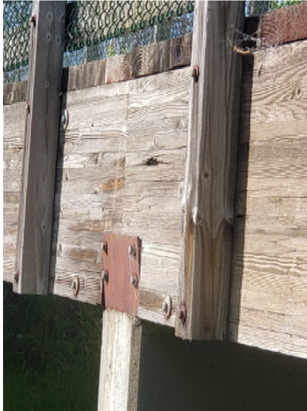
Image 11: Center Girder Splice
