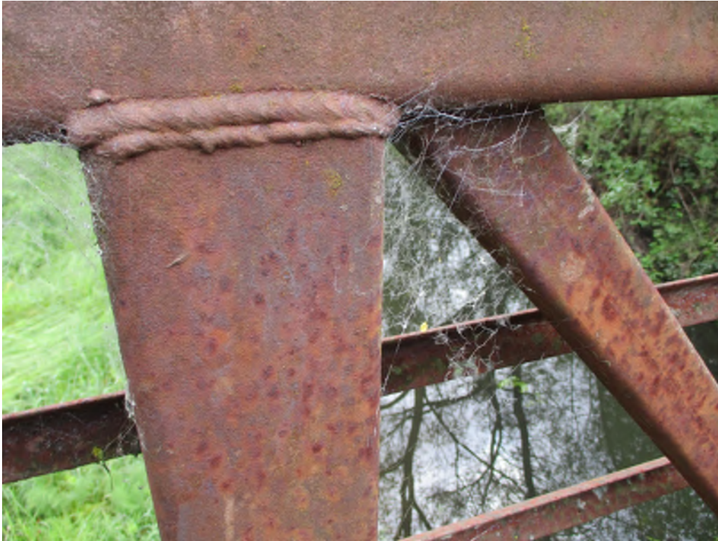
Image 5: Truss Typical Brace/Post Top Connection
