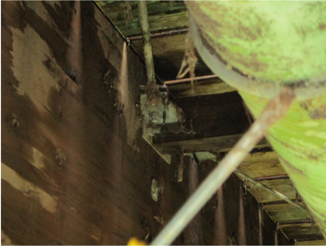
Image 13: Lateral Bracing
