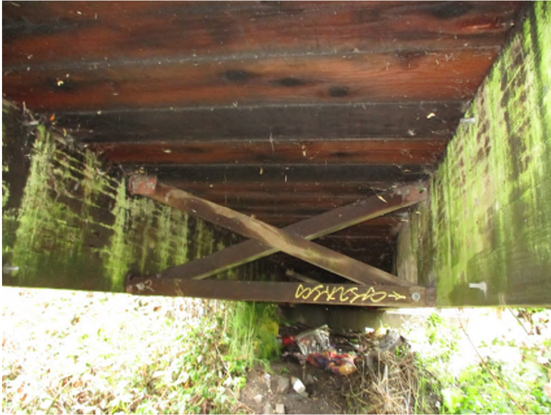
Image 11: Underside of Bridge
