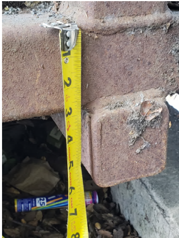
Image 12: Gravity Purlin Connection
