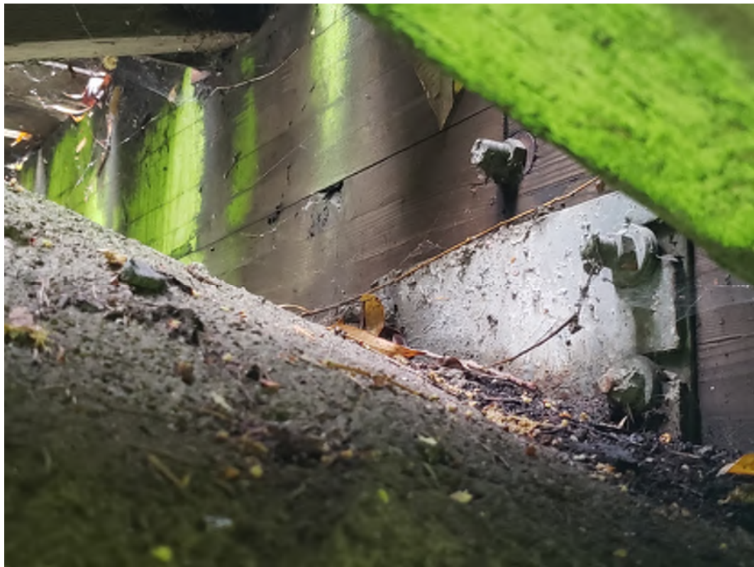
Image 14: Internal Bracket at Center Splice
