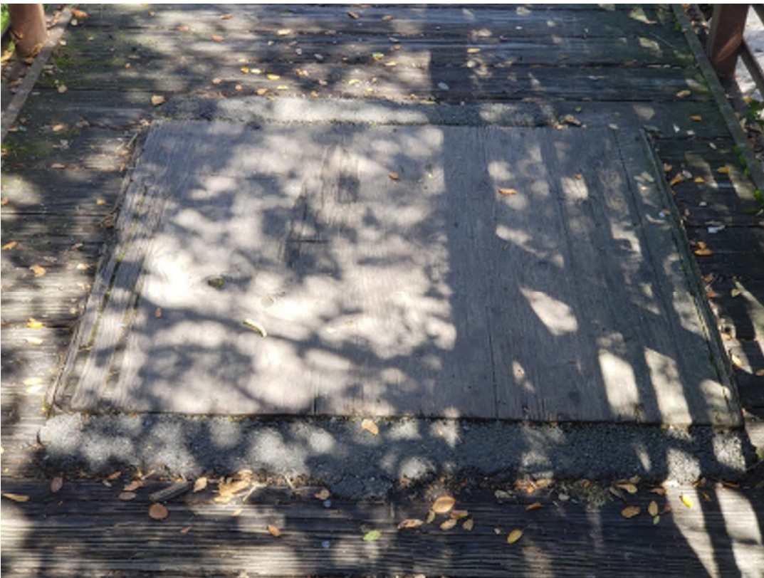
Image 8: Floorboard Patch
