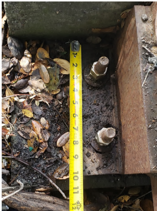
Image 10: Typical Bearing Plate and Anchor Bolt
