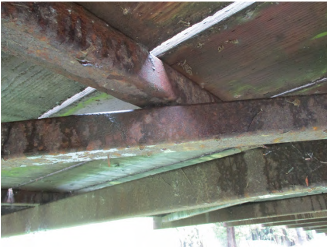
Image 14: Horizontal Bracing under Gravity Framing
