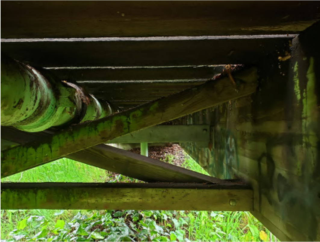
Image 13: Underside of Bridge
