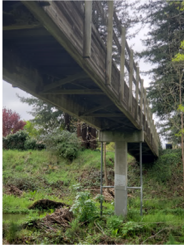
Image 13: Underside of Bridge
