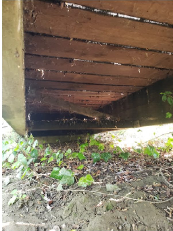
Image 11: Underside of Bridge
