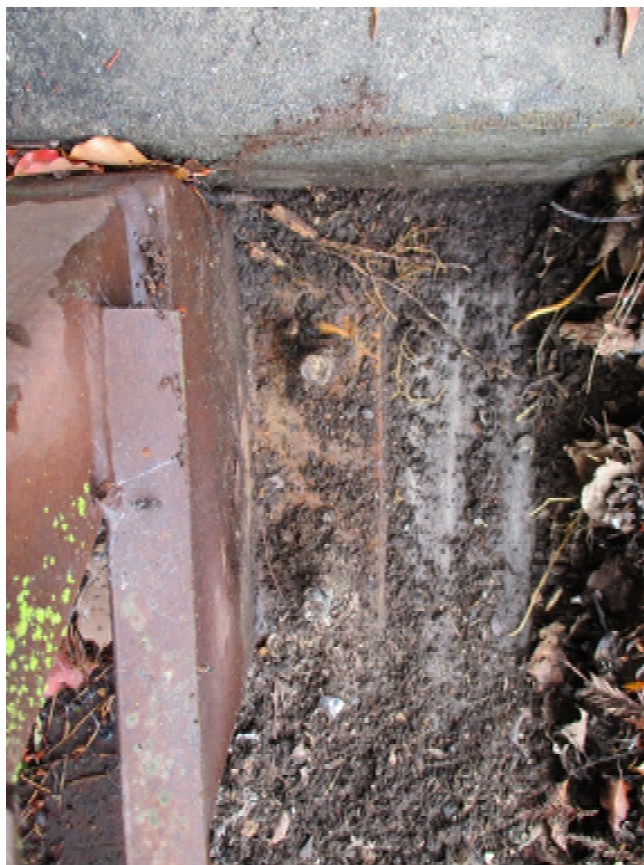
Image 10: Typical Bearing Plate and Anchor Bolt
