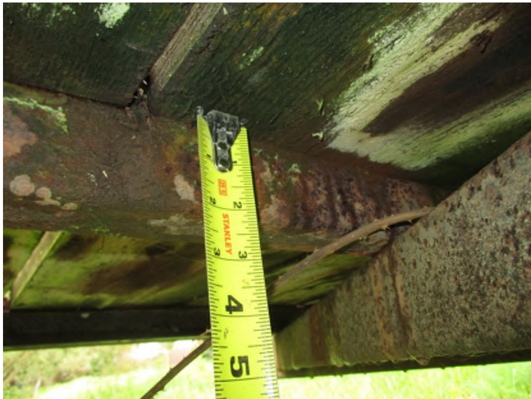
Image 14: Horizontal Bracing under Gravity Framing
