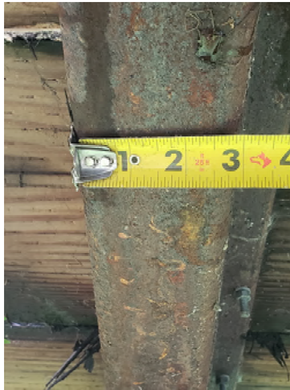
Image 11: Floorboard Gravity Framing
