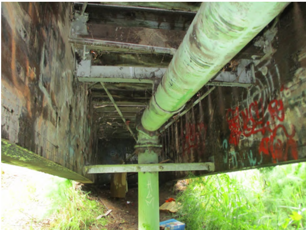
Image 12: Underside of Bridge
