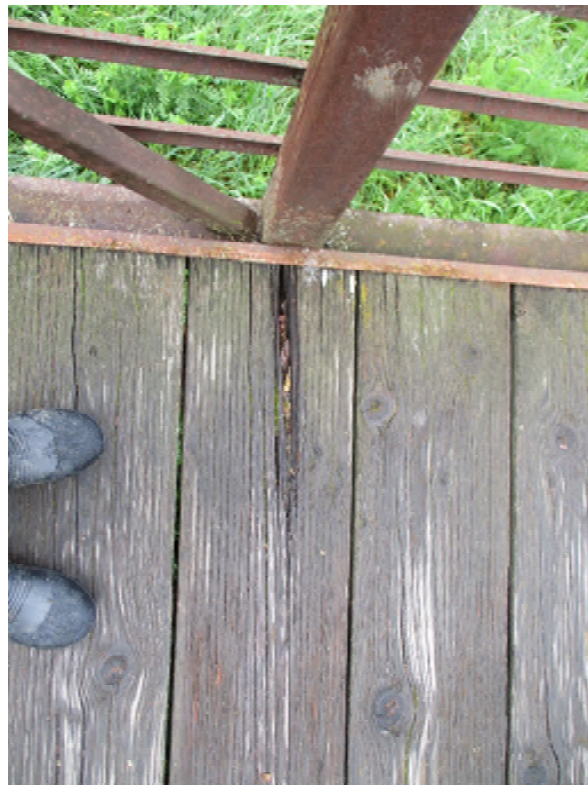
Image 6: Truss Typical Brace/Post Bottom Connection
