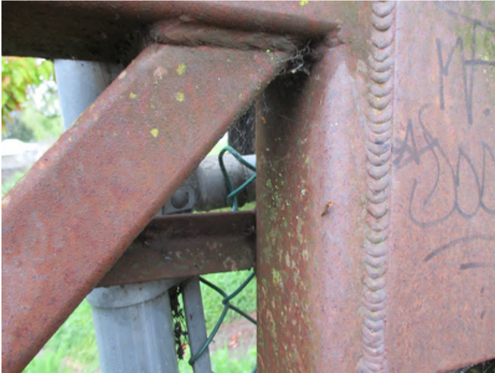
Image 5: Truss Typical Brace/Post Top Connection
