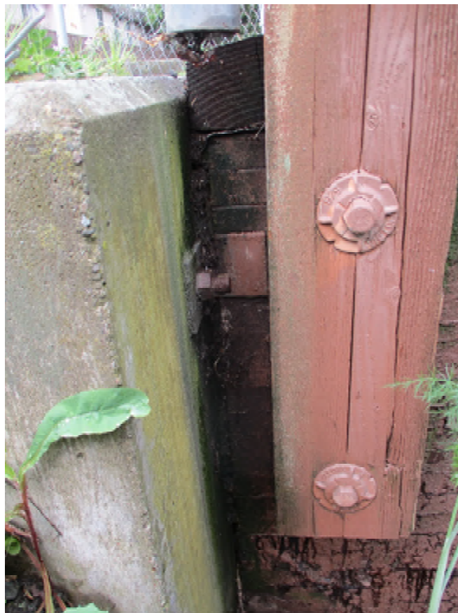
Image 6: Handrail Post Connection
