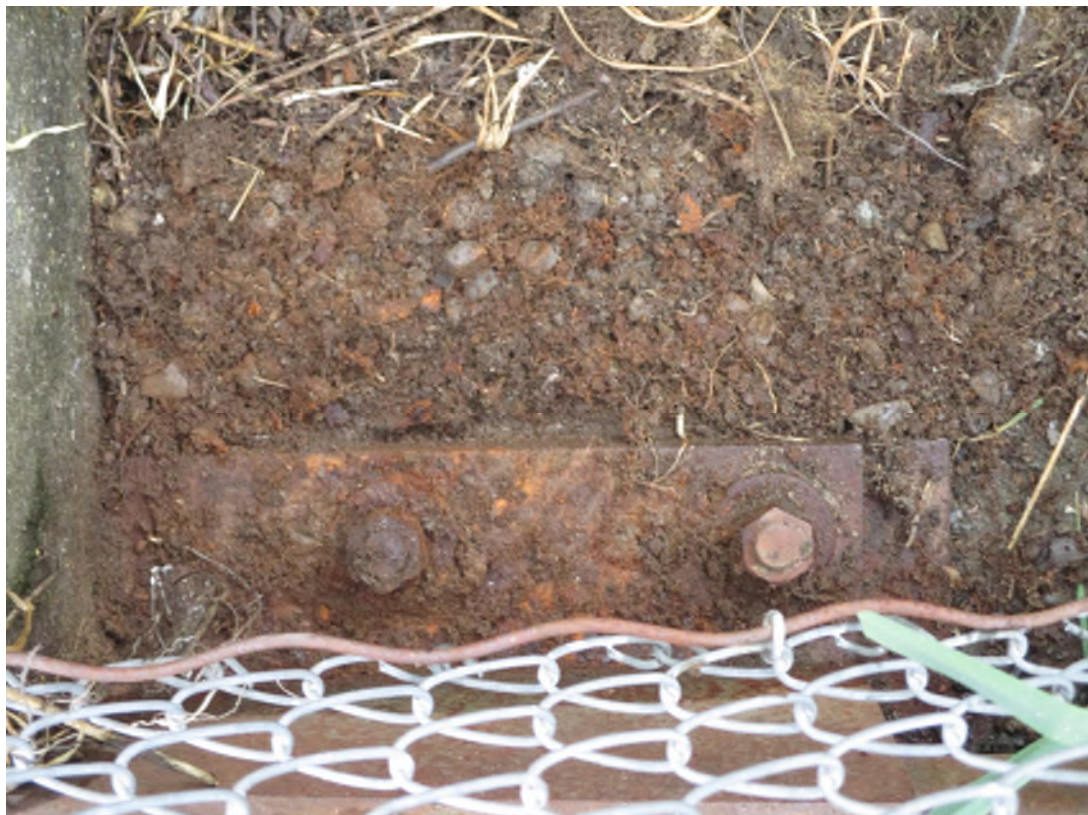
Image 10: Typical Bearing Plate and Anchor Bolt
