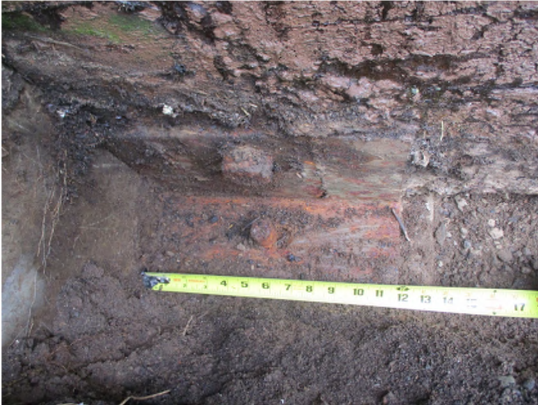
Image 9: Typical Bearing Plate and Anchor Bolt
