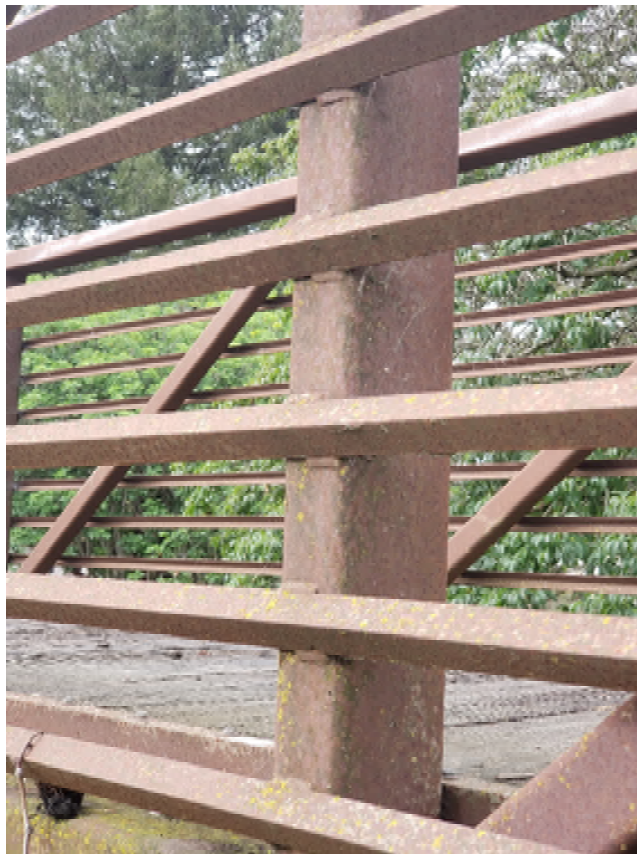
Image 6: Typical Handrail Member Weld
