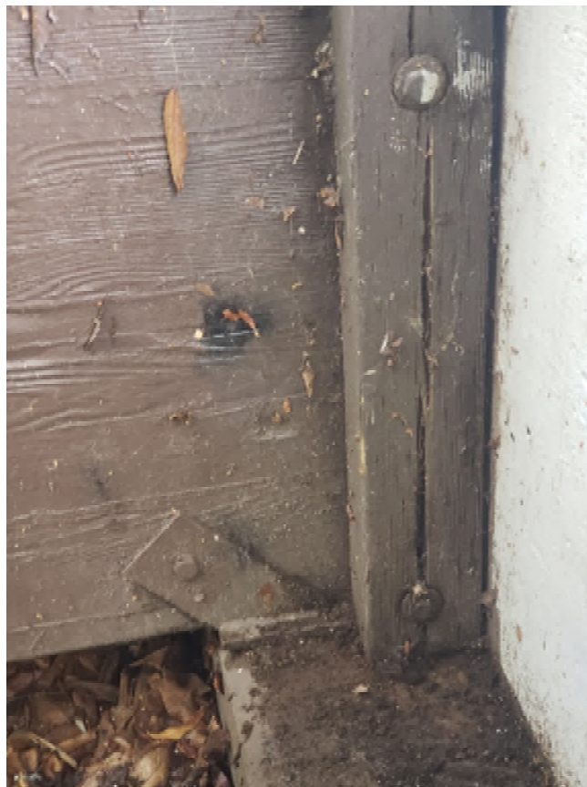
Image 10: Typical Bearing Plate and Anchor Bolt
