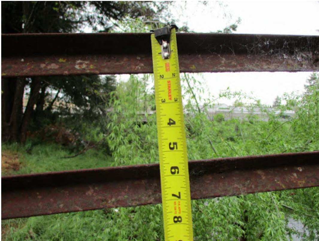
Image 15: Maximum Horizontal Member Spacing
